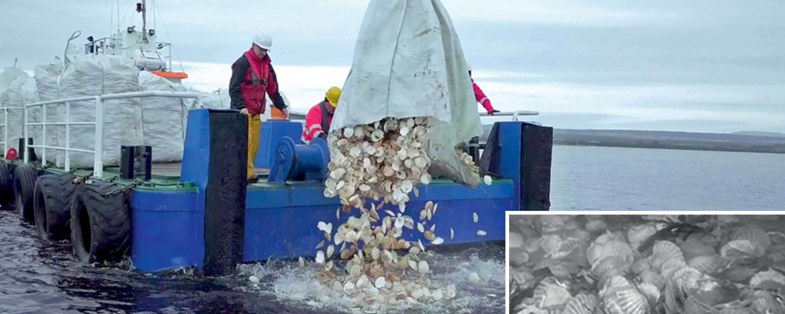
**Figure 3.8:** The deployment of shell (cultch) from bags off the bow of a barge in the Dornoch Firth, Scotland. This method allows the shell to fall at one time and form a more consolidated mound on the seabed. Photo: Jean Paul.
